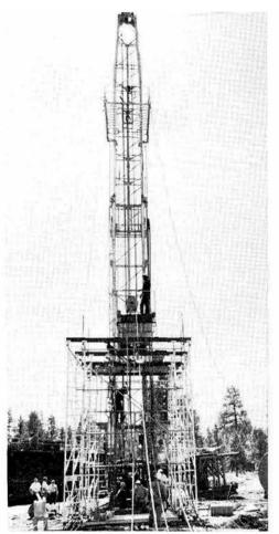
HEAVY DUTY CABLES-16,000 feet of itrun from remote recording trailer and down the drill hole to the buried Sandia seismic instruments. The Gasbuggy site is in the Carson National Forest, 50 air miles from Farmington.
